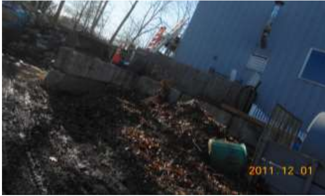
Figure 2 Property very muddy, poor drainage and erosion.
